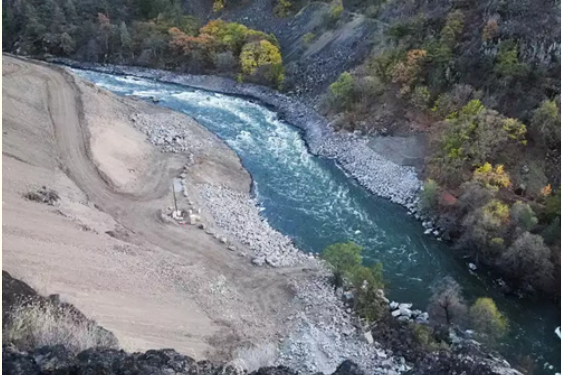
Copco No. 2 After
