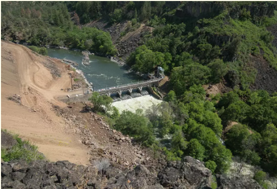
Copco No. 2 Before
