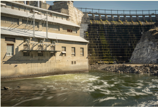
Copco No. 1 Before
